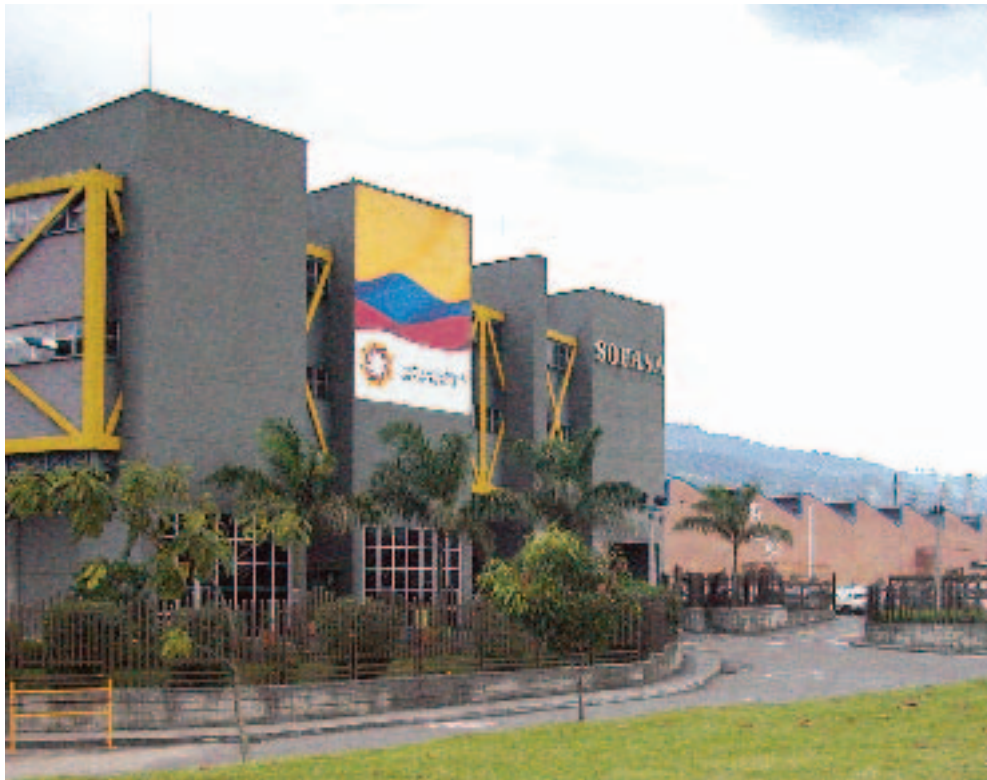
The L90 will be assembled by Sofasa in Colombia.
