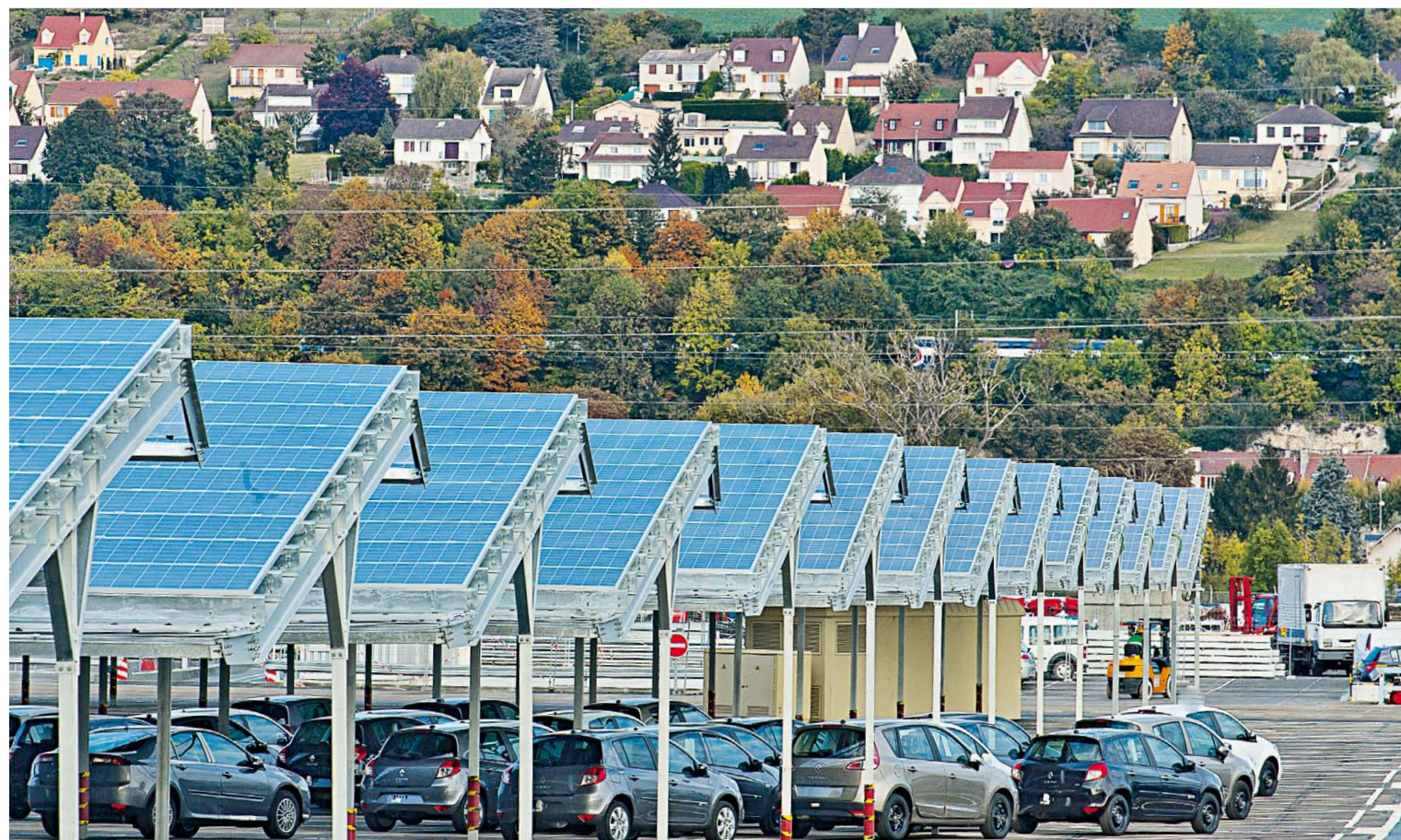
Renault has launched the world's biggest photovoltaic project in the automotive sector, with 450,000 m 2 of solar panels on the roofs our French plants. Here, the Flins plant.
