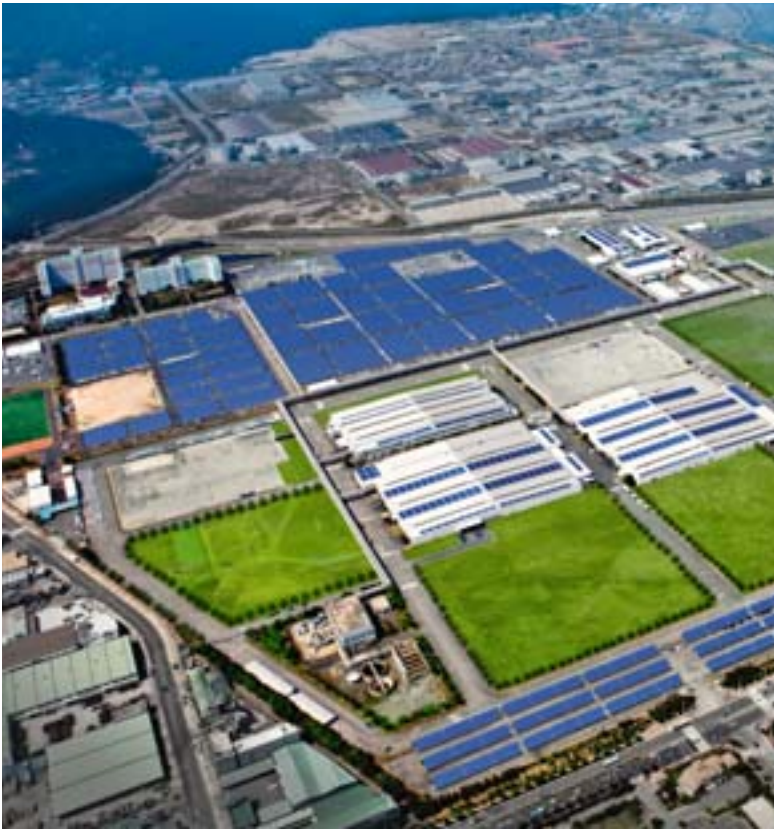
Solar panels at the RSM plant in South Korea: this is the largest such installation in the world at an industrial site.
